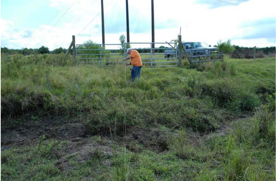
Looking south at existing upland cut, intermittently flowing irrigation ditch.
