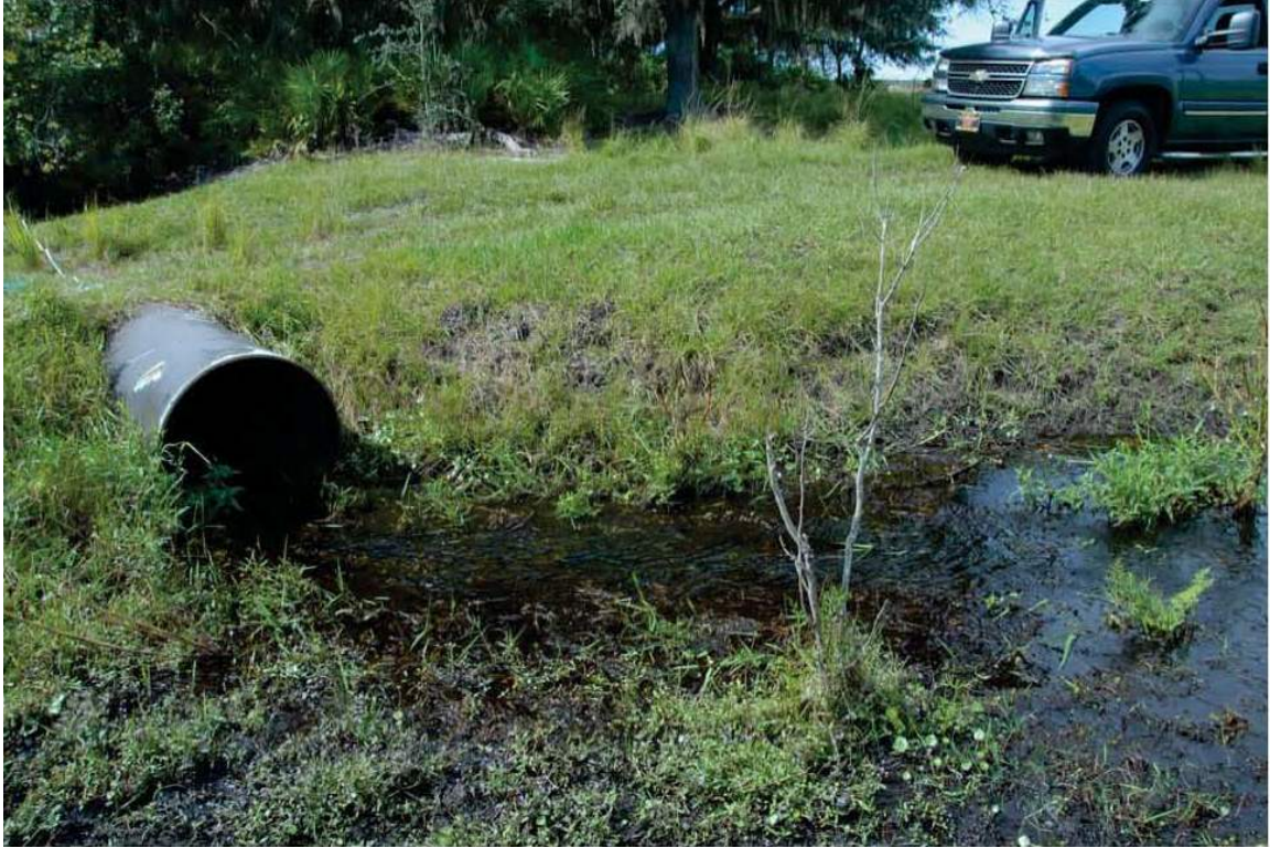
Looking east at the upstream end of the existing culvert.
