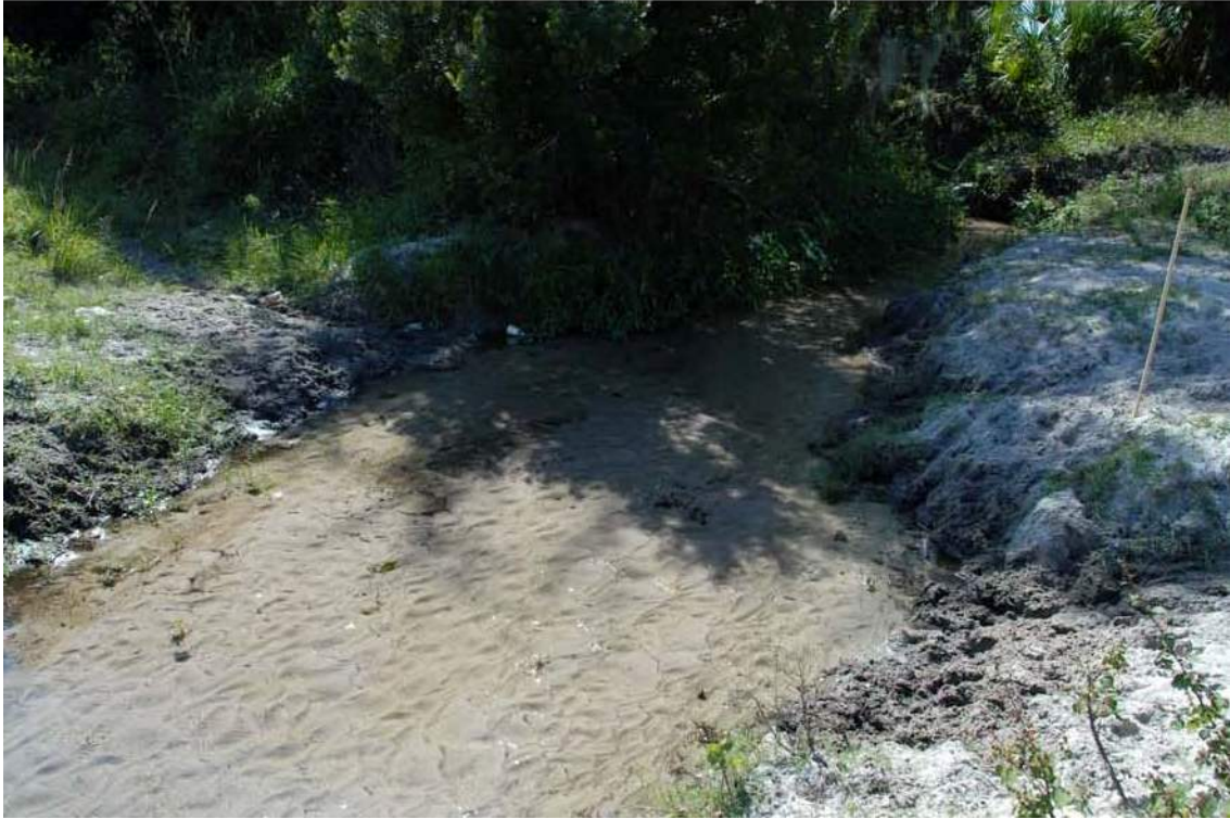
Looking east at upstream end of existing low water crossing showing mostly non-vegetated banks with resultant erosion. Note non-native bahia grass on left side of photo and Caesar's weed on lower right portion of the photo.
