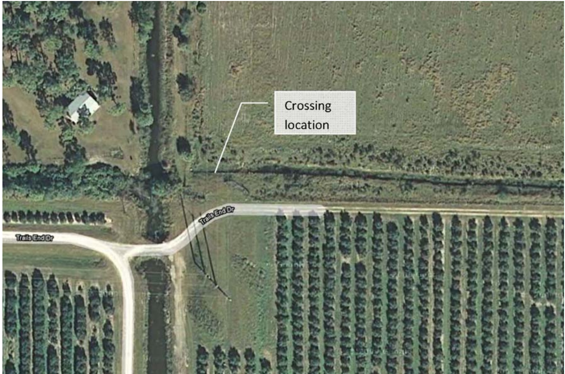
Drainage Crossing between Structures 301 and 302 – Photographs.
