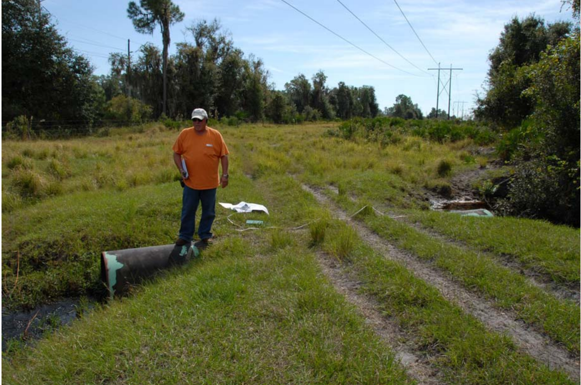
Looking south at the existing 30-inch culvert.
