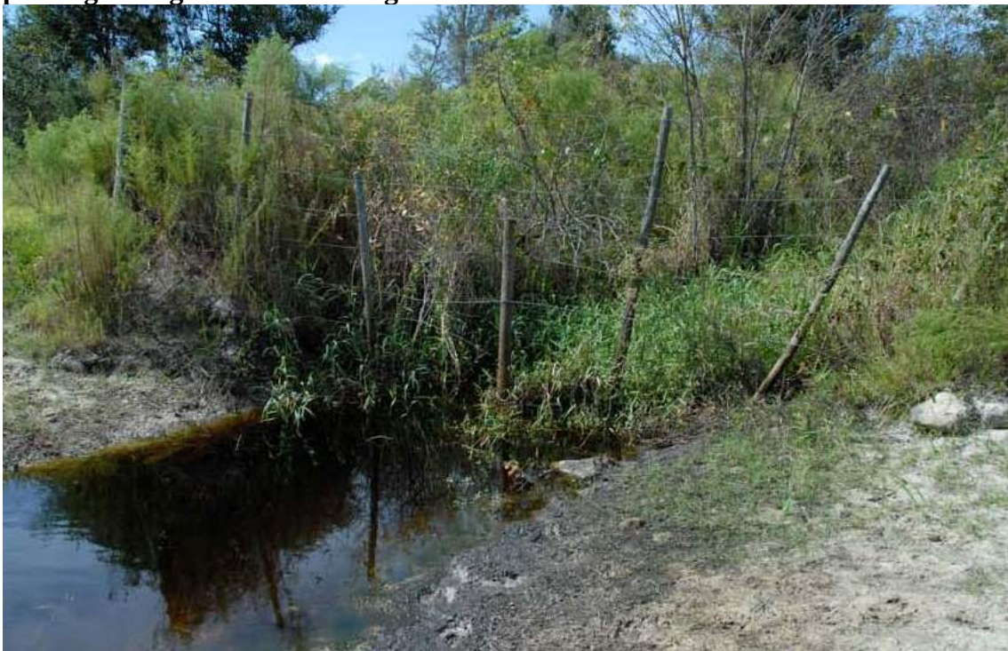
Looking west at upstream end of low water crossing.
