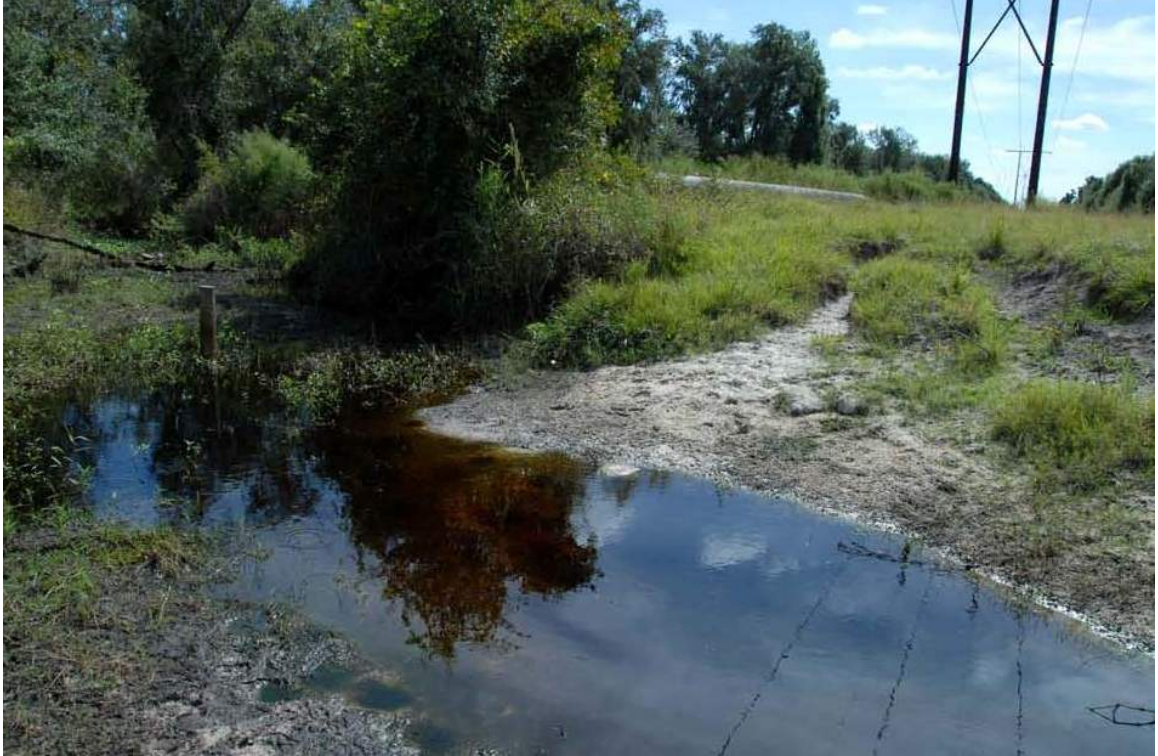
Looking southeast at downstream end of low water crossing showing cattle impacts.
