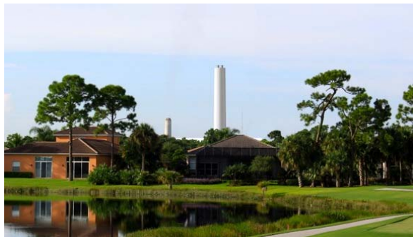
Figure B-4 Conventional stack from north
