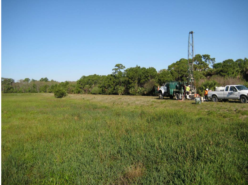
Photograph 5: Drilling rig located on Boring TB-10, viewing west.
