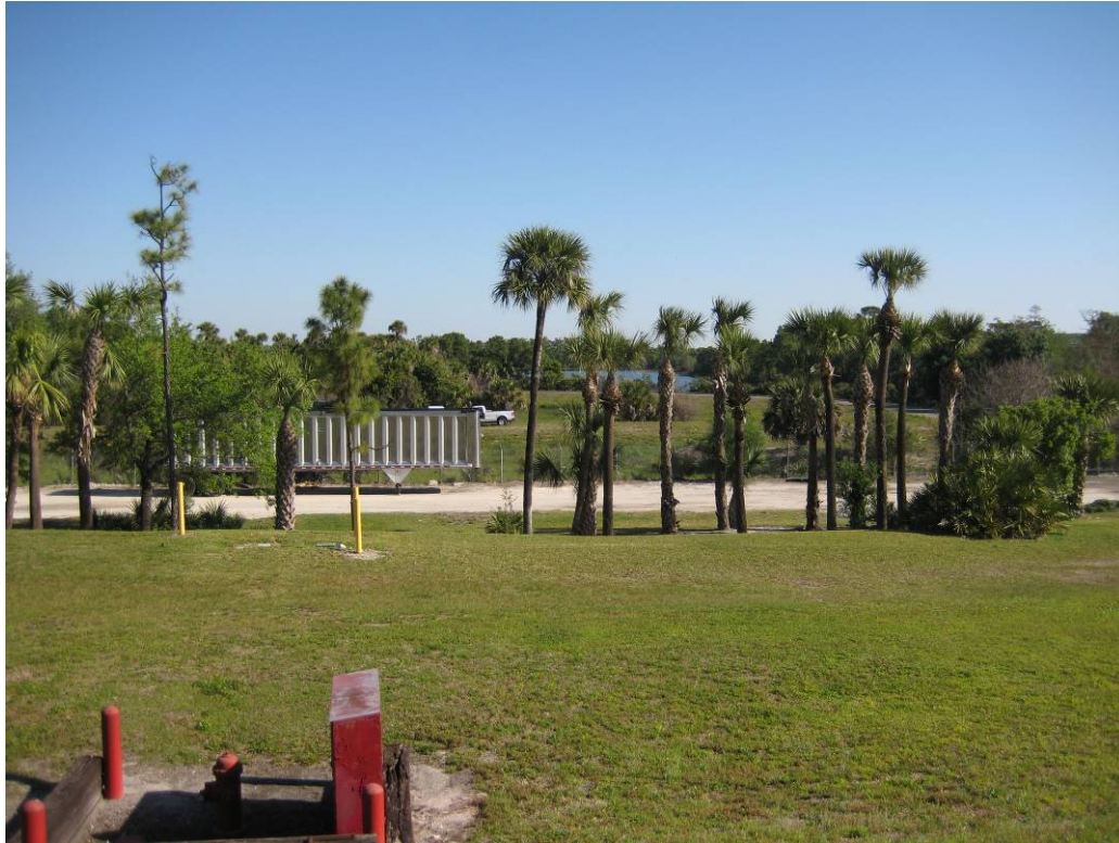
Photograph 3: Site viewed north from near NE Corner of existing facility.
