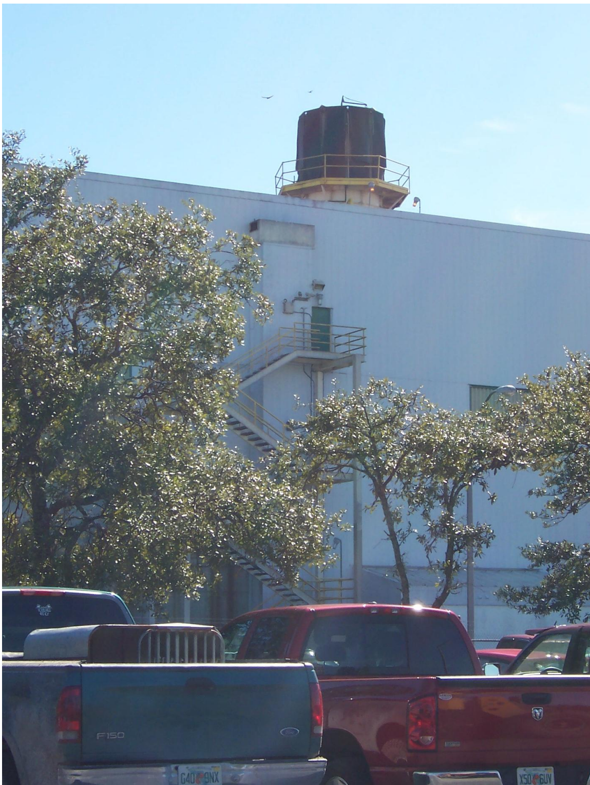
Figure 4-2: OBW Shredder Vent
