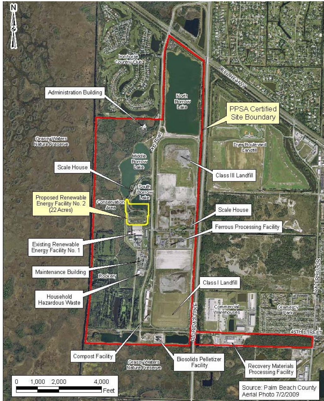
Figure 2-2: Facilities at the Palm Beach Renewable Energy Park
