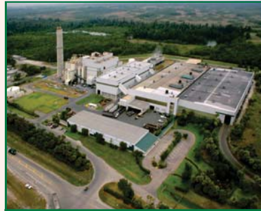
THE EXISTING NCRRF ON JOG ROAD.
