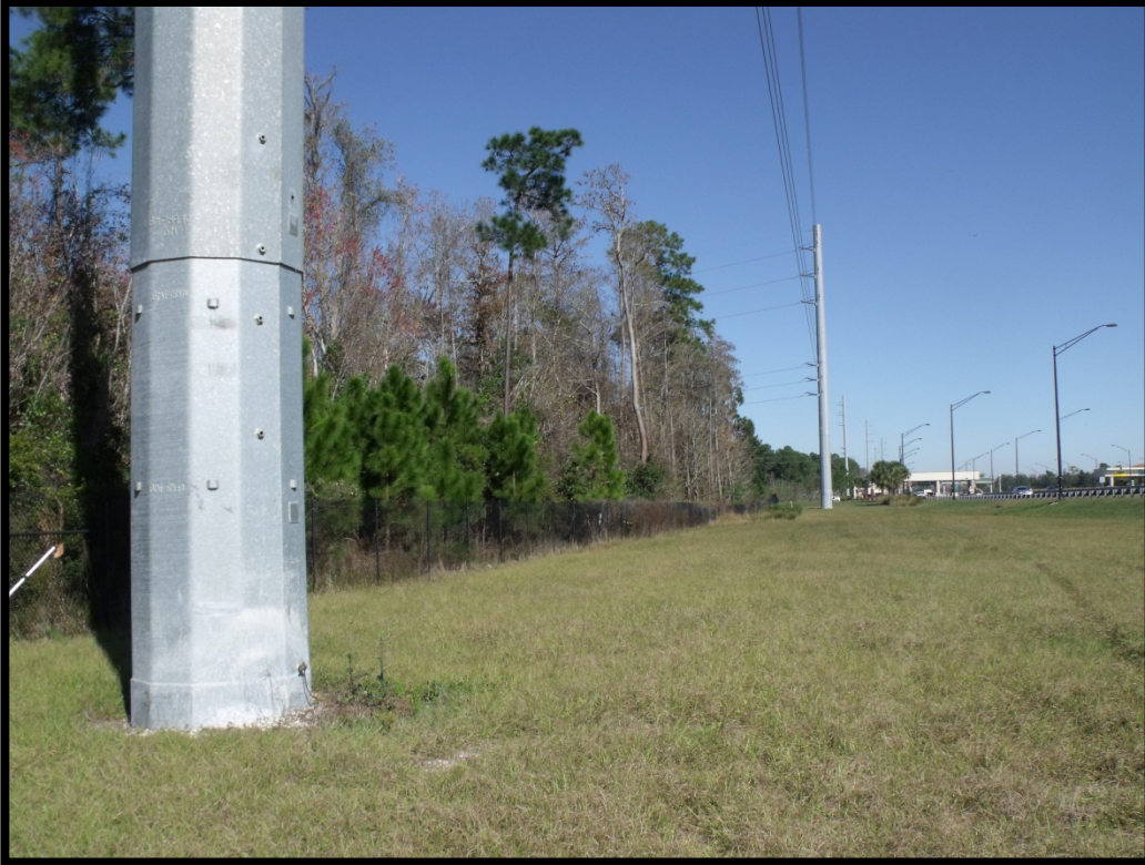
Photo Point 45 – Wetland WL-32, view looking north.
