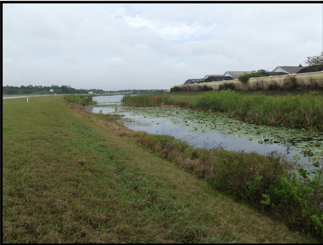
Photo Point 26 – Surface Water SW-5, view to the north.
