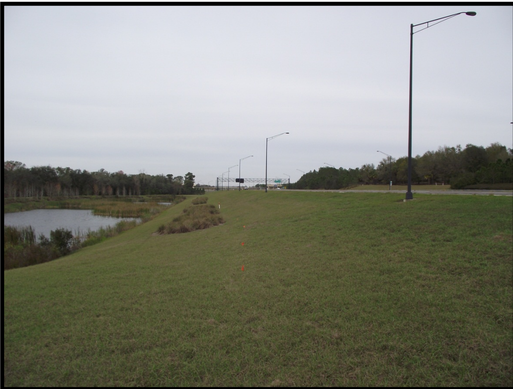
Photo Point 4 - View of the SR429 right-of-way from proposed structure ICG-47 looking north.
