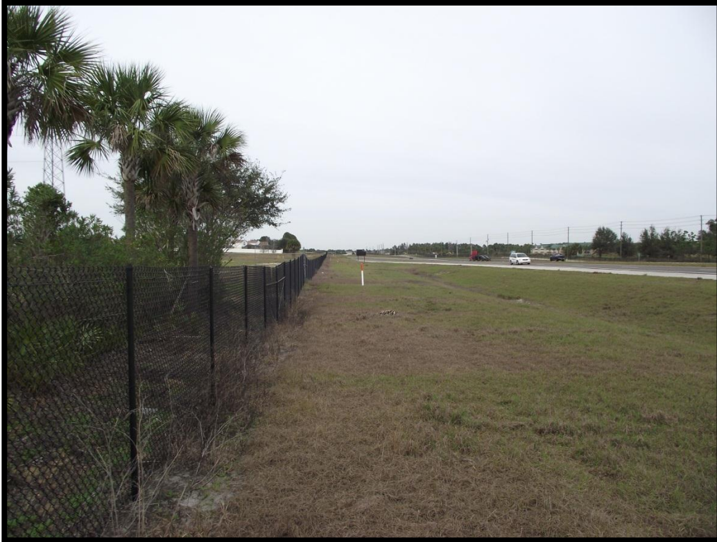
Photo Point 19 – View of FDOT right-of-way, looking north, in front of the Water treatment plant.
