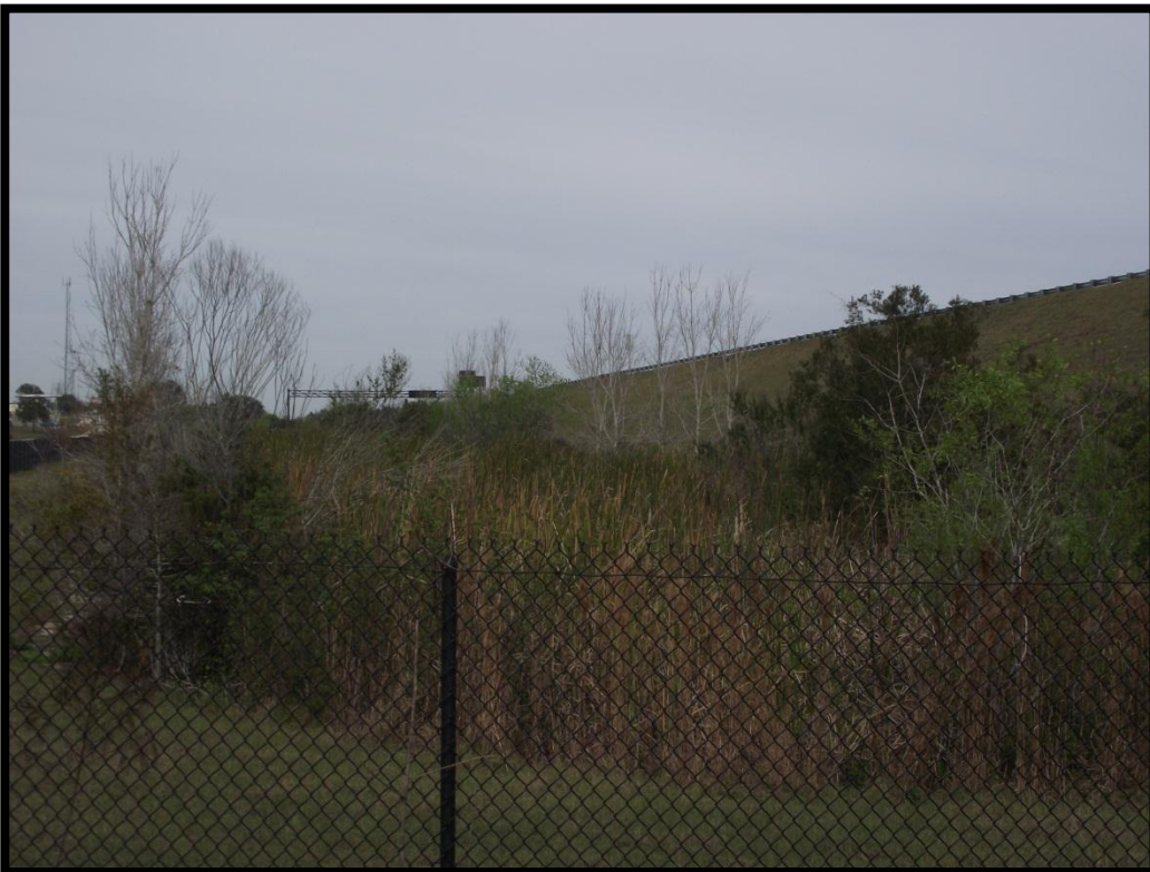
Photo Point 18 – Surface Water SW-2, stormwater retention pond, view to the north.
