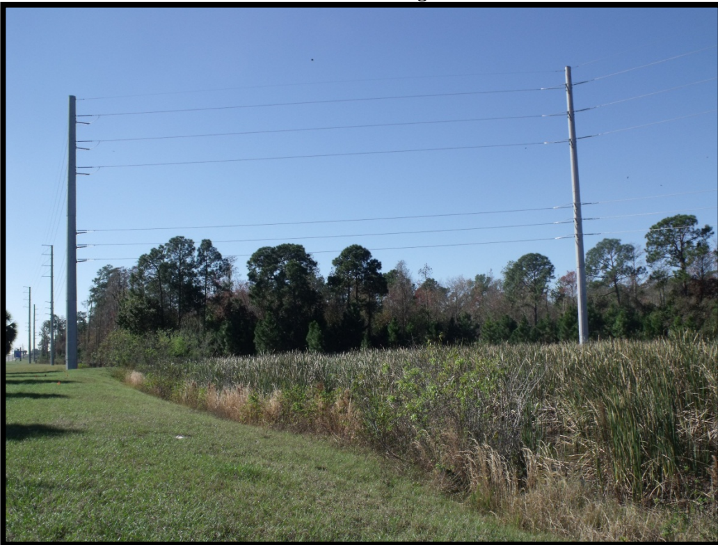
Photo Point 46 – Surface Water SW-13, looking southwest.
