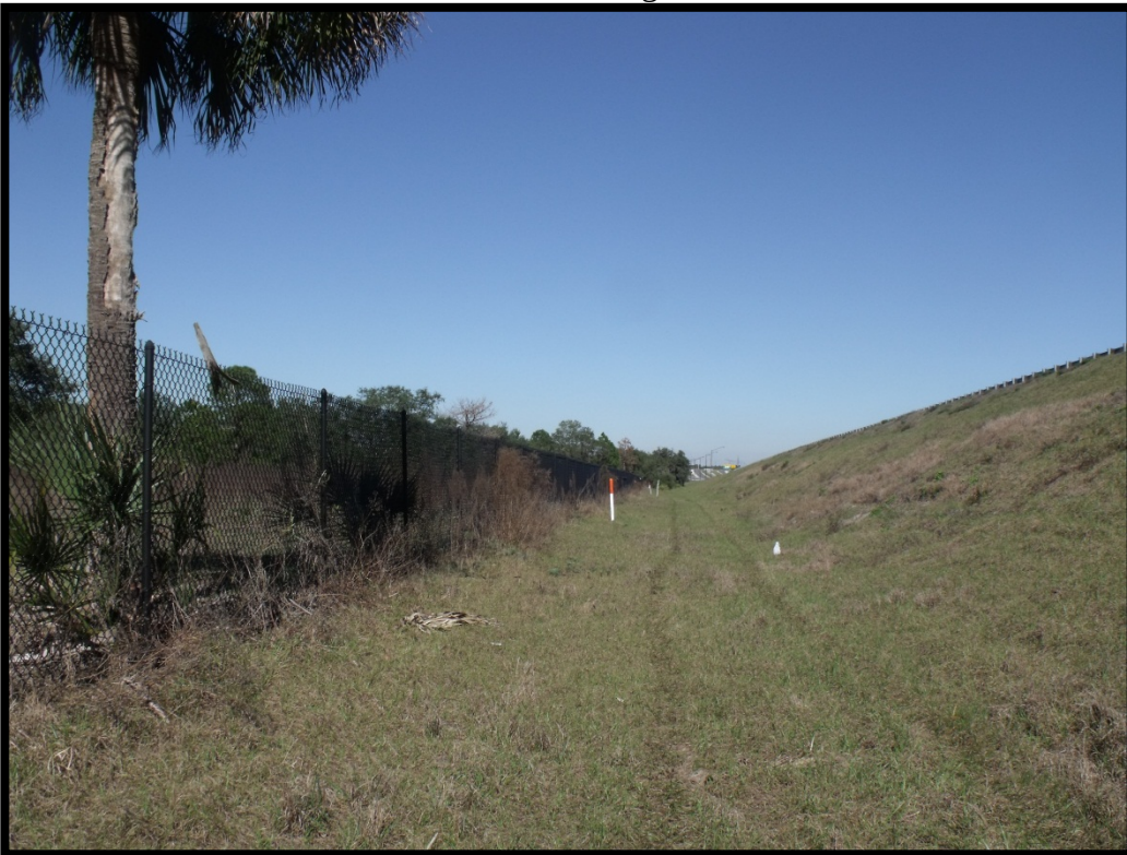
Photo Point 30 – View of upland area, looking north from proposed structure ICG-81.
