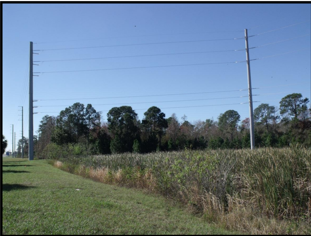
Photo Point 46 – Surface Water SW-13, looking southwest.
