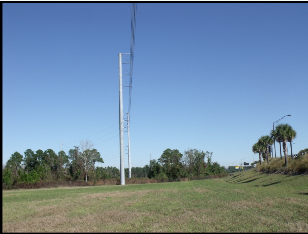
Photo Point 40 – View looking north from proposed structure ICG-91.
