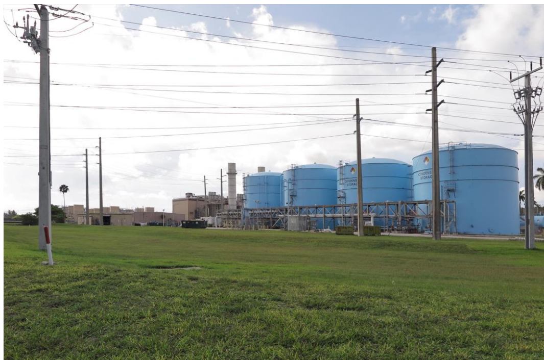
Figure 11. Project parcel looking east from a point east of South New River Canal (8BD4153 – behind photographer) across temporary construction laydown area.
