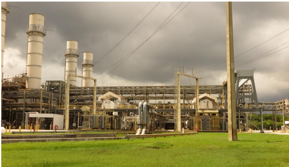
Figure 23. 8BD6078, Steam Turbine Units 4 and 5, looking south.
