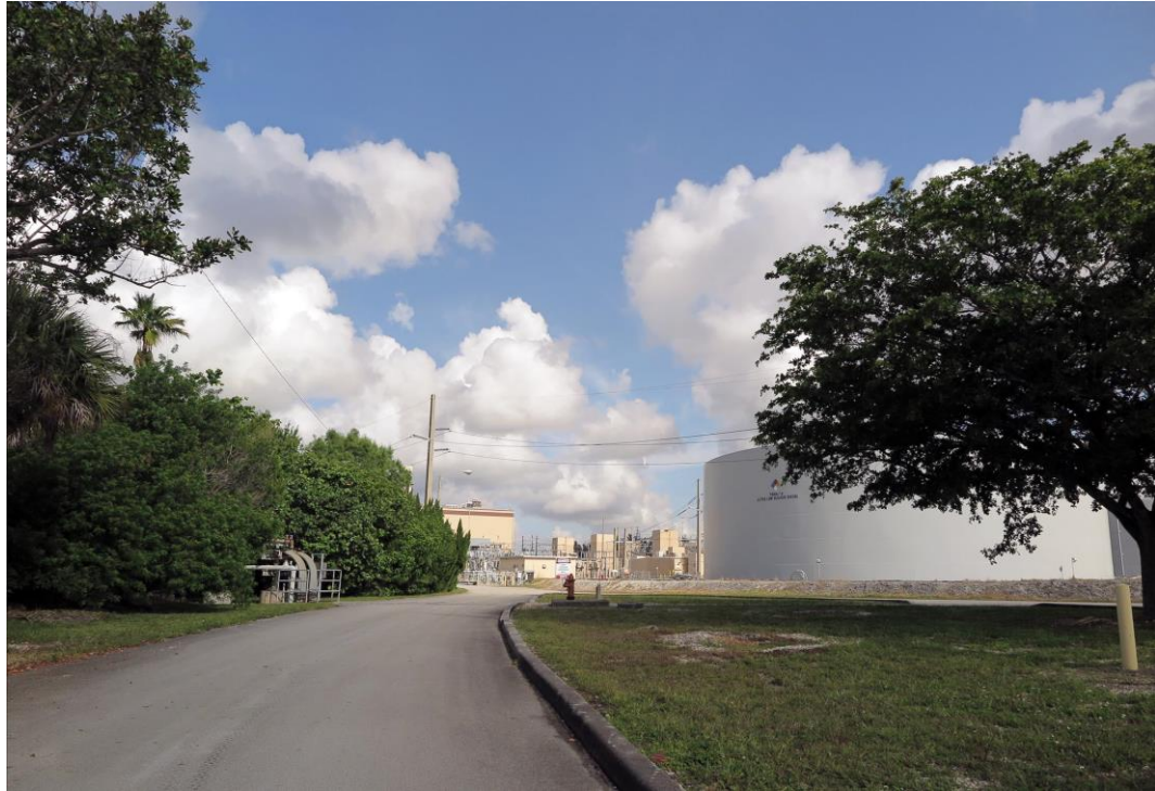
Figure 14. Project parcel looking northwest from southeast corner of property across temporary construction laydown areas (left and right of road.)
