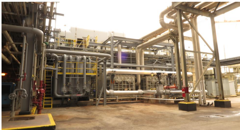
Figure 24. 8BD6078 looking west, buried in equipment, barely visible.
