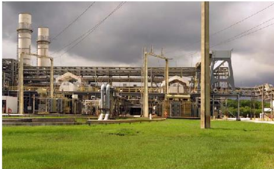
BD6078 (tan painted cylindrical equipment under gabled roofing) looking south, 6/16/17.
