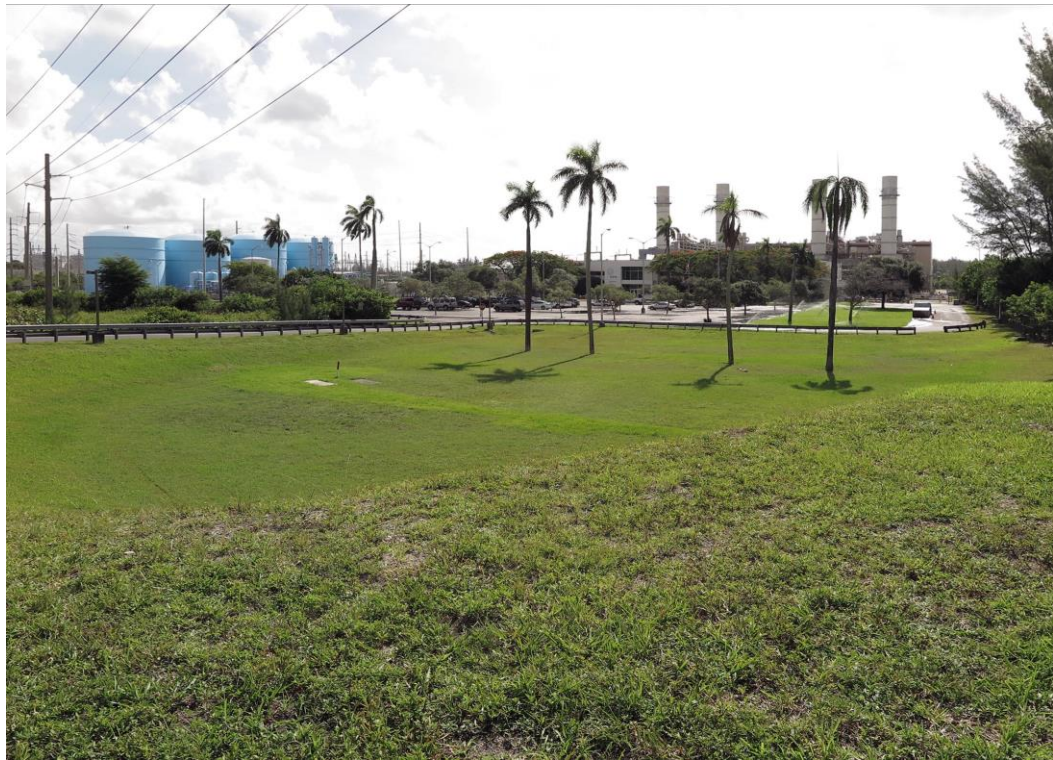
Figure 10. Project parcel looking north across temporary construction laydown area of from southeast corner of property; entrance at bridge over Dania Cut-Off Canal (8BD3221 – out of photo to right). Area proposed for new construction is visible on right horizon.
