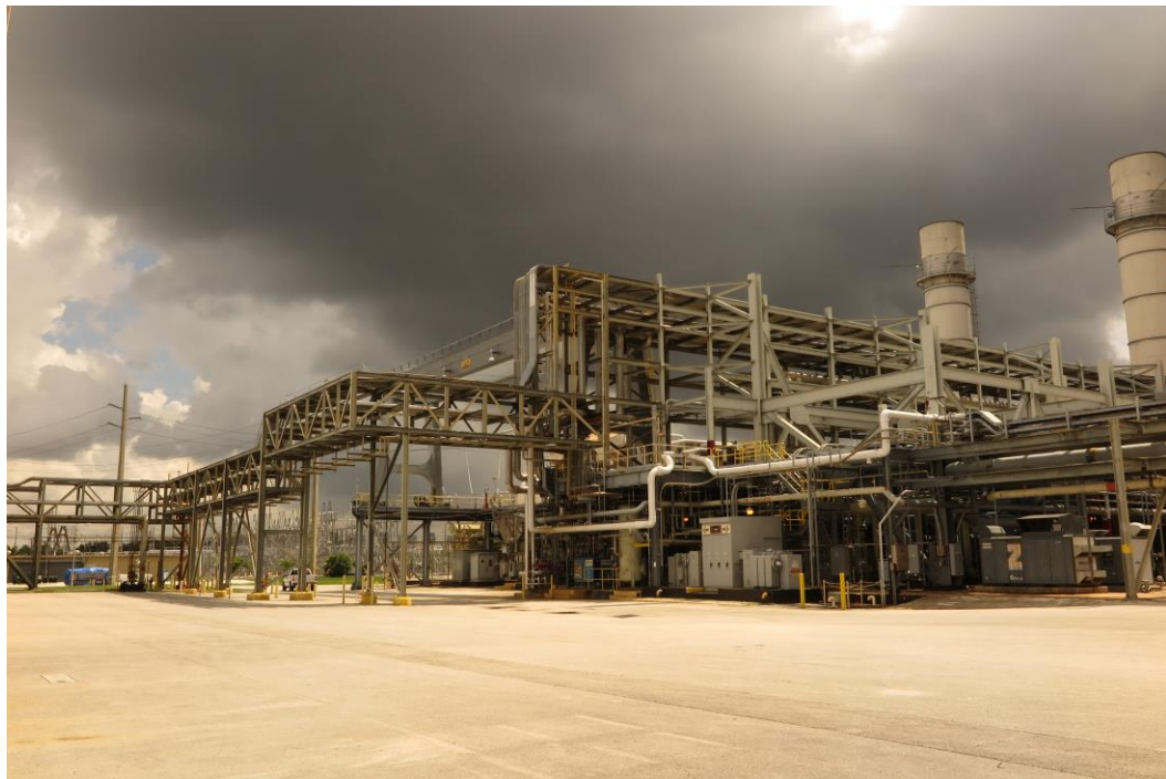
Figure 15. Looking northwest at existing plant (proposed for new construction.)
