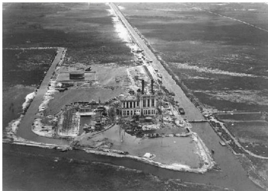
Aerial view looking east of 1926 flood with FPL Lauderdale newly constructed. BD4153 turns north where BD3221 cuts off to the east. The Dania Cut-Off Canal was the primary conveyance for supplies during construction of the power plant, leaving the main canal relatively untouched (photo: FPL archives).
