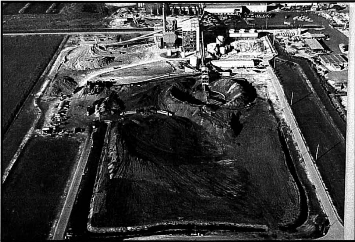
Figure 3.2-3a. NHPP Wood and Bagasse storage and handling.
