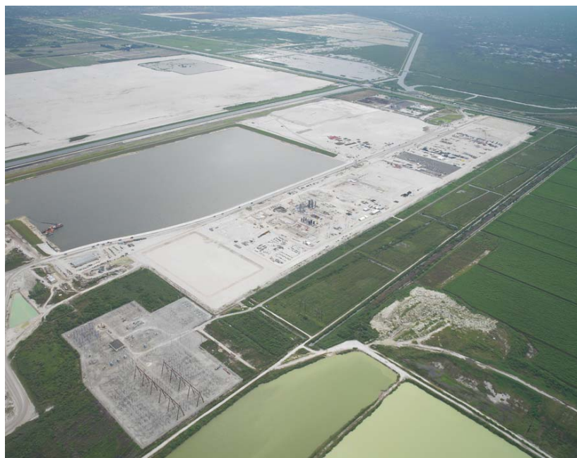
Figure 2.1.0-5. WCEC Site showing Units 1 and 2 under construction. View from northwest to southeast.
