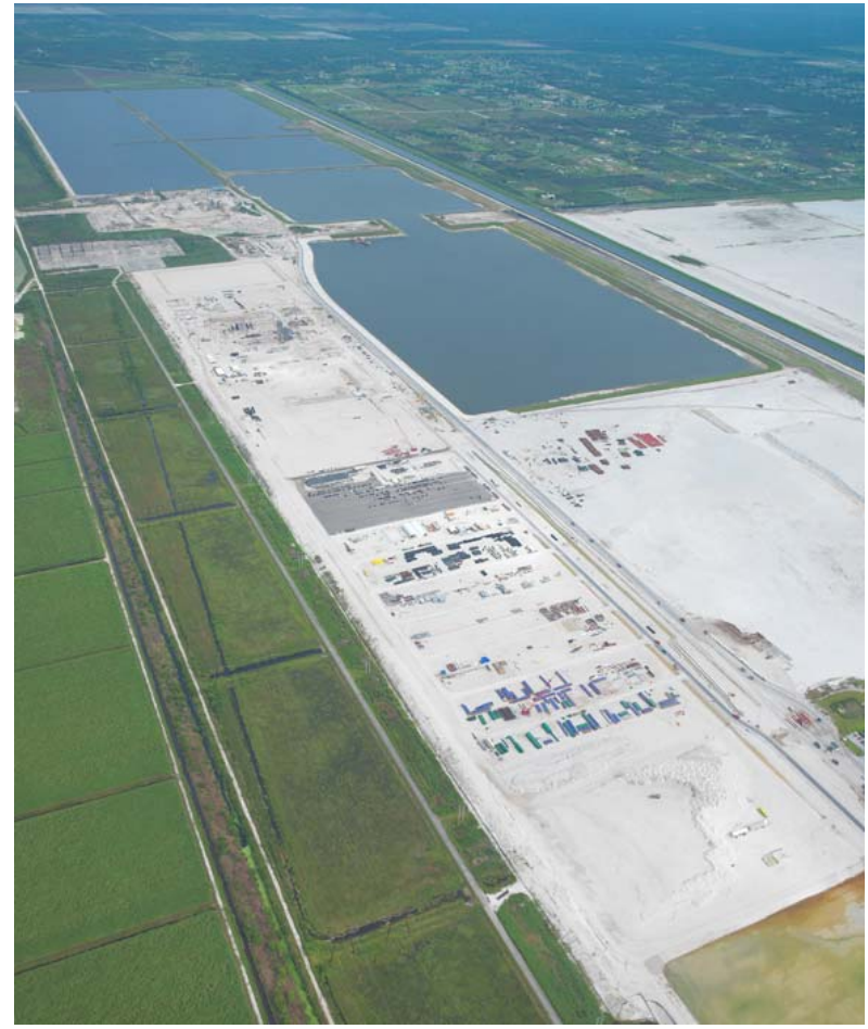
Figure 2.1.0-3. WCEC Site showing Units 1 and 2 under construction. View from southwest to northeast.
