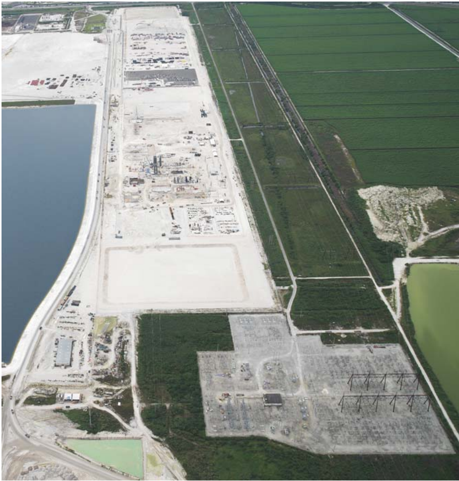
Figure 2.1.0-2. WCEC Site showing Units 1 and 2 under construction. View from the north to the south.
