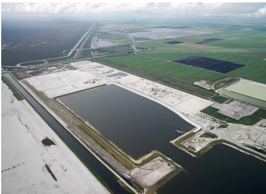
Figure 2.1.0-4. WCEC Site showing Units 1 and 2 under construction. View from northeast to southwest.
